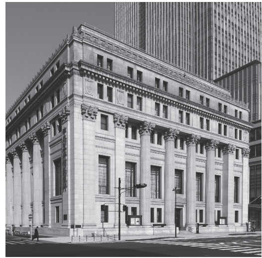
Fig.3 現在の三井本館と超高層 Present Mitsui Main Building and Nihombashi Mitsui Tower
