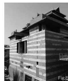
Fig.5 ひろしまハウス外観 Hiroshima House: Outside view Fig.6 ひろしまハウス内部 Hiroshima House: Inside view
