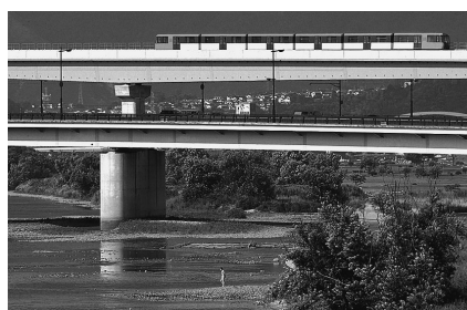
Fig.5 太田川中流域、新交通システムが走る New transportation system running across the River Ota at its middle course.
