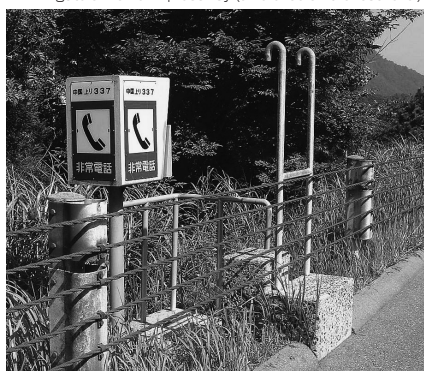
Fig.7 中国道下り安佐SA付近の電話（ワイヤ跨ぎ必要） Telephone near the Asa Interchange on the down line of Chugoku Expressway (Users have to step over the cable.)
