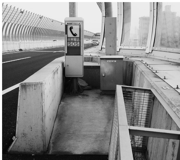
Fig.9 東名阪道の平田IC付近の電話（スロープ式） Telephone near the Hirata Interchange on Higashi-Meihan Expressway (Slope)
