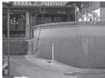
Fig.2 避難誘導灯 Evacuation light
